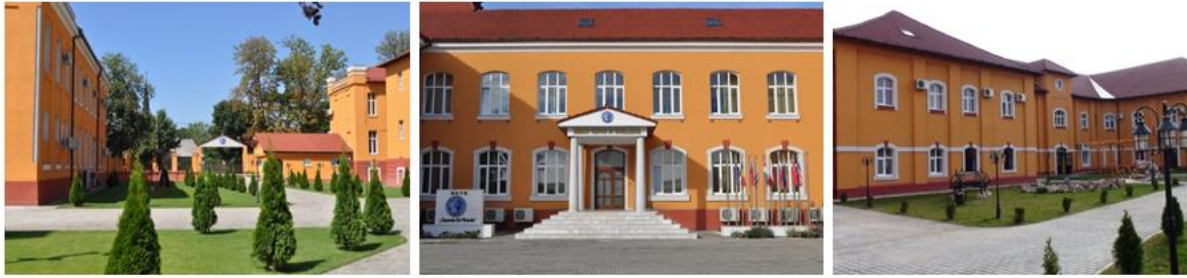
Fig.2 The NATO HCOE – internal view
